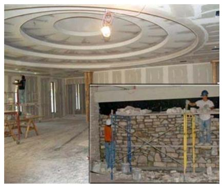
The photograph above shows construction workers working on the sheet rock in the Reading Room and on the Limestone wall surrounding the exterior of the building.
