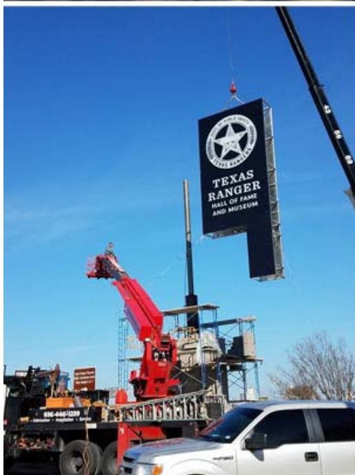
Top: Monument sign on truck bed being delivered to the site. Middle Left: Large cranes are used to place monument on the center support rod. It is then welded into place. Middle Right: Limestone is wrapped around the cinder block center to complete the monument. Below Left: Ground level monument is placed on cinder block core and wrapped with limestone. Below Right: Finishing the monument with silver aluminum edging.
